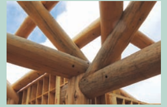
Corner detail—the level of complexity achieved by Nininger and his crew.
