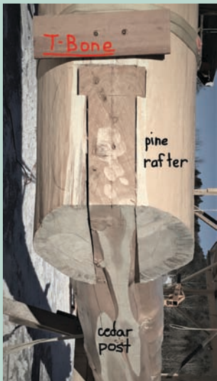
T-bone: This T-shaped tenon and mortise secures the truss to the upright both laterally and longitudinally.
