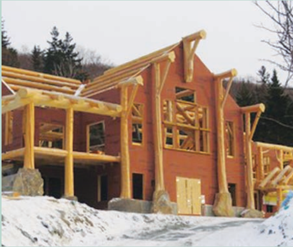
Exterior: Front of Lodge under construction.
